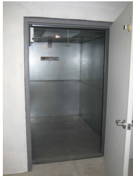
The VRC carriage is lighted and covered with reflective diamond-plate wall and floor panels that enhance illumination and protect property from damage. The durable ArmorCar carriage interior never requires painting.
